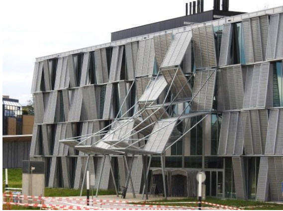
Fig.12: ME Building (Laboratory of Biomaterials) in EPFL Campus in Lausanne, Switzerland. It is an example of emphasizing the entrance approach by the design of a kinetic canopy, designed by Dominique Perrault Architecture - Source: Photographed by the author, 2019
